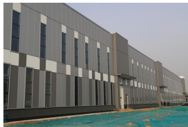
vertical installation of exterior wall panels
