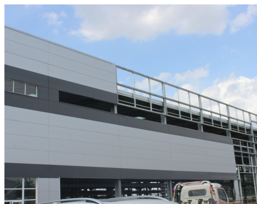
Horizontal installation of exterior wall panels
